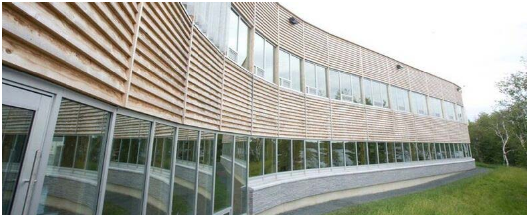
Figure 2.3: Wood siding and stone cladding shown on the Living with Lakes building. Obtained from Laurentian University Office of Sustainability.
