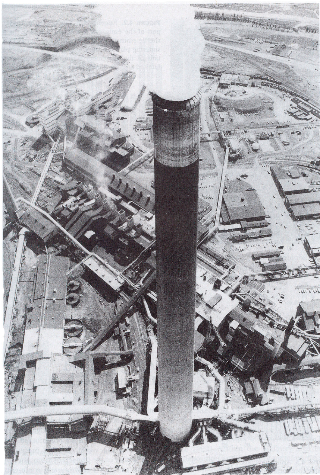
FIGURE 4.1. Inco Limited Superstack (Sudbury Star Files) constructed in 1972 to reduce local impacts of industrial emissions. Technologies at Inco to reduce the quantity of pollutants released into the atmosphere are described in Chapter 21.
